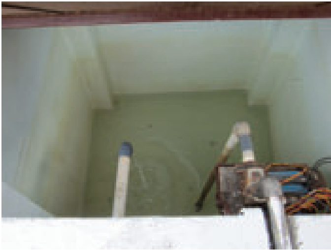
Collection tank of treated wastewater
