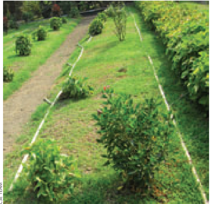
SBT gravel trench and bioreactor
