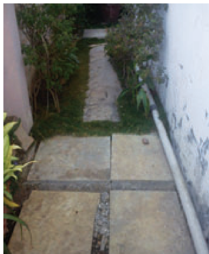
Piping and equalisation tanks
