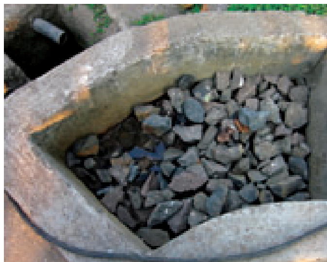
Inlet zone with filter media
