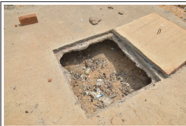
Incineration ash dumping pit at RIMS, Ranchi
