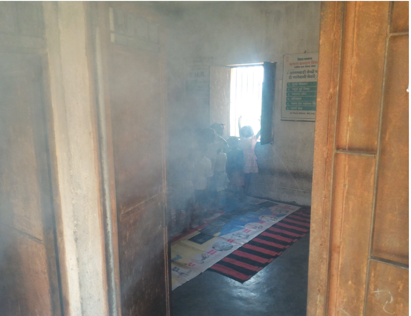
Improperly ventilated rooms are quickly filled with smoke which remains trapped with the children for at least two hours
