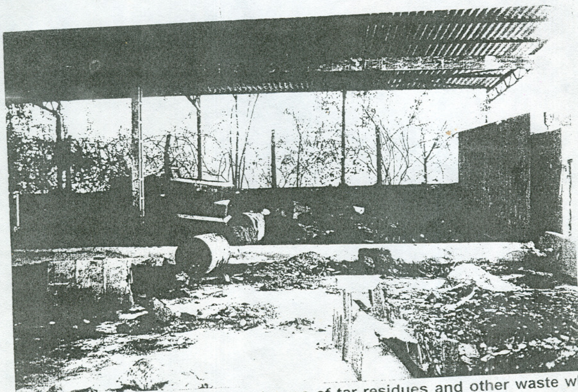
PLATE 1 : Photograph showing storage of tar residues in a shed (earlier used to be a cycle stand). Polythene bags were found torn-off and drums corroded
