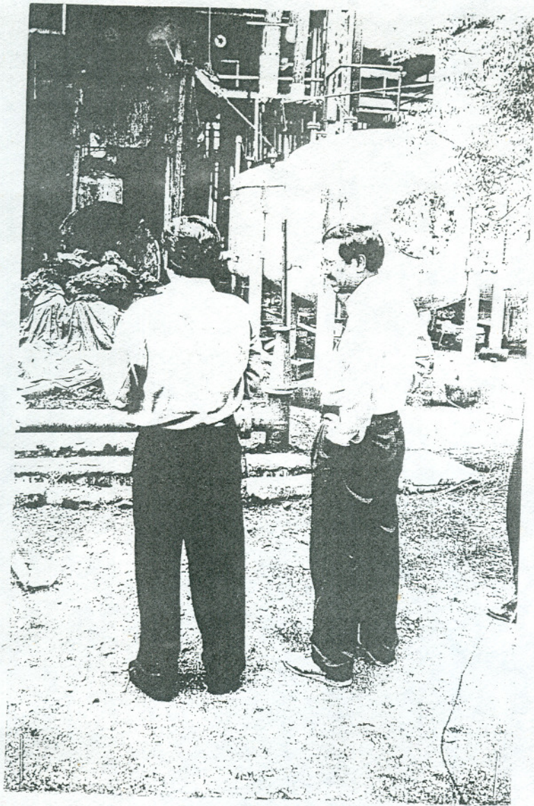
PLATE 3 : Photograph showing collapsed reactor and hazardous material spread on the floor of the plant, the run-off which is likely to find way into the storm water drain
