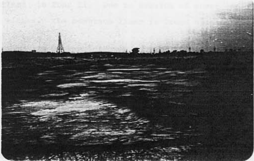
SOLAR EVAPORATION POND II SHOWING EXPOSED MEMBRANE LINER
