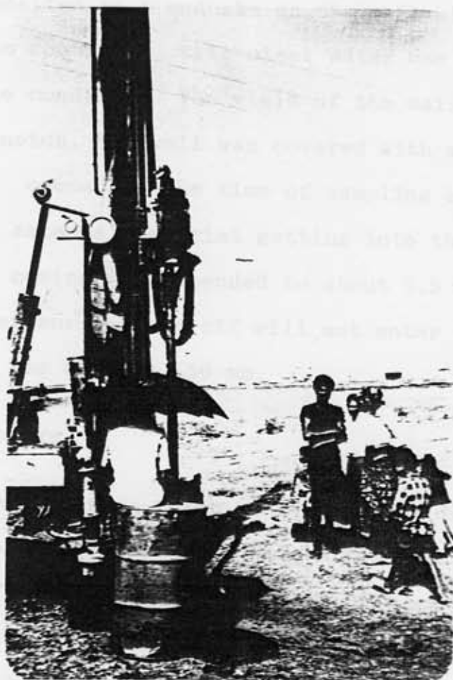
DRILLING OF A TEST BORE WELL
