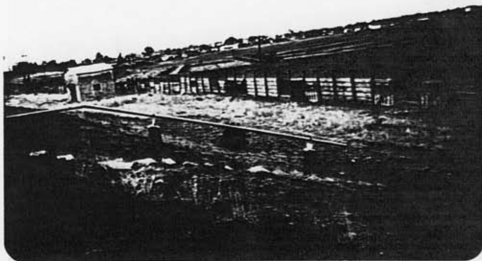
WASTEWATER INLET PIPE TO SEP
