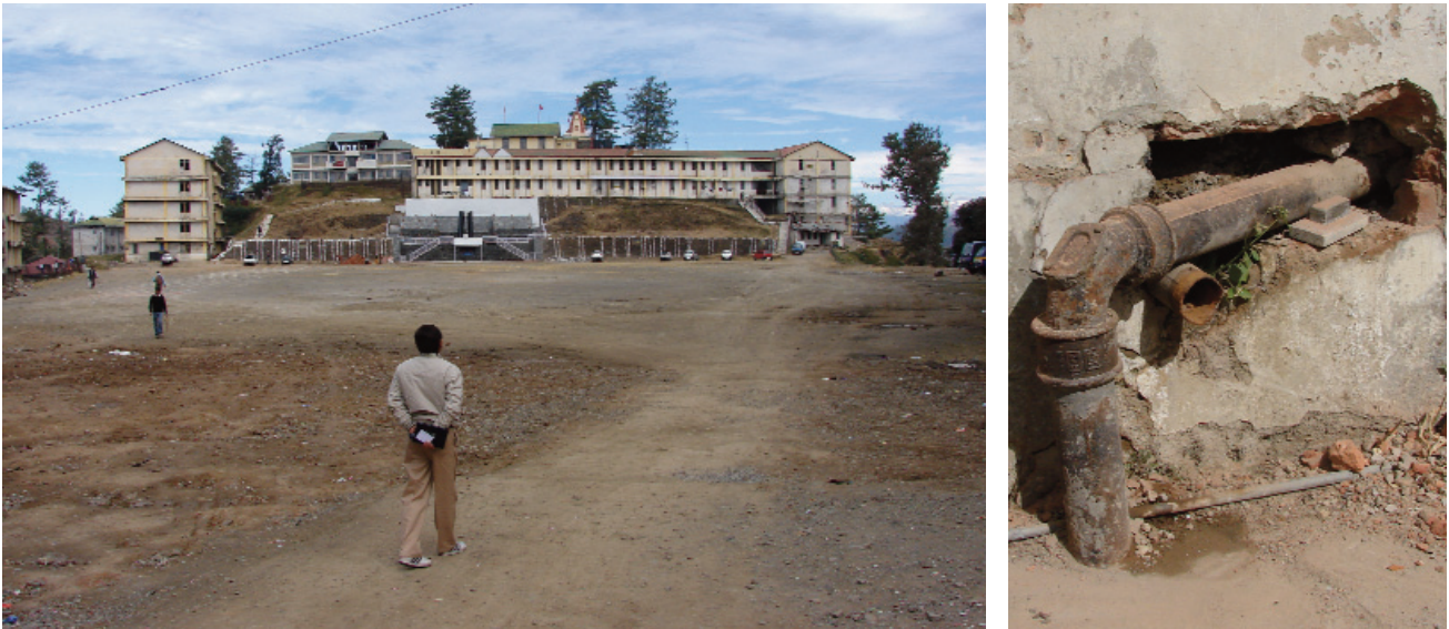
Picture 4 (a) Police Ground at Bharari (b) pipeline connection to septic tank
