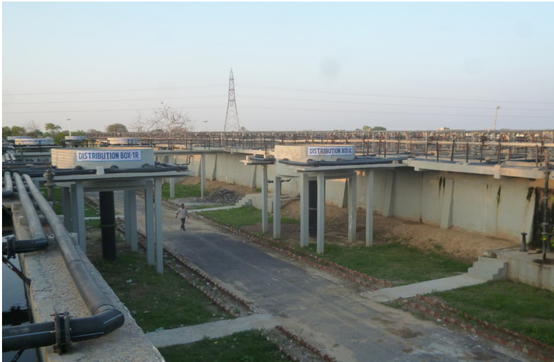
Figure 5: 78 MLD UASB technology Dhandpura STP (Source: Shantanu/CSE, 2015)
