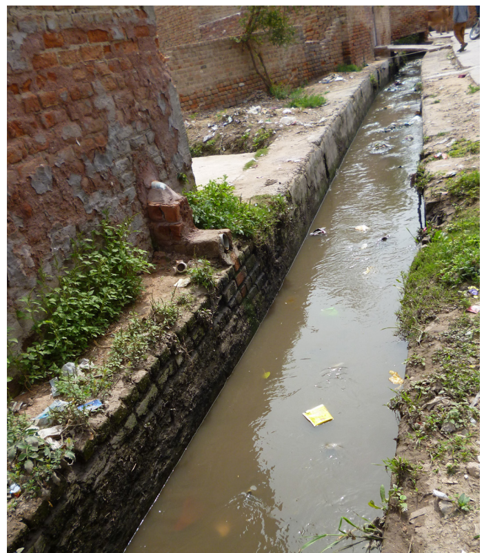
Figure 1: WC to open drains (Source: Shantanu & Rahul/CSE, 2015)
