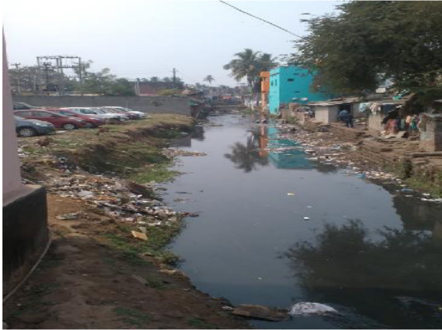
Figure 3: Open drain carrying sewage (Source: Shantanu/CSE, 2015)
