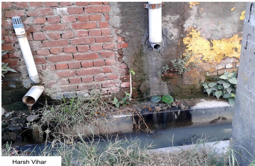
Septic tank connected to open drain
