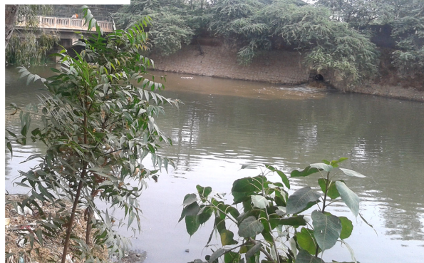
Sewage disposal into nullah
