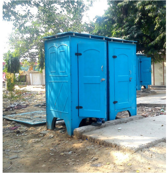
Figure 22: Prefabricated bio-digester toilets in night shelters (Source: Anil/CSE, 2015)
