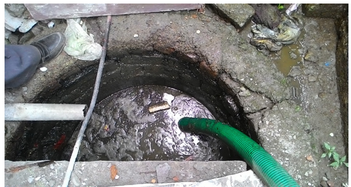
Figure 1: Emptying from chambers (Source: Rahul/CSE, 2015)
