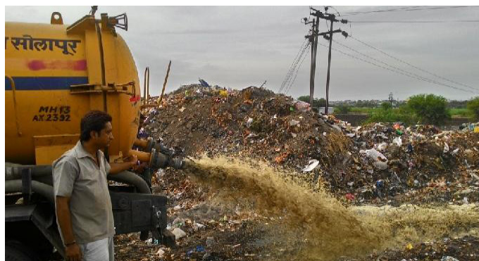
Figure 3: Disposal of septage in solid waste dump yard (Source: Rahul/CSE, 2015)
