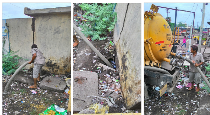
Figure 1: Emptying process of septage from community toilet (Source: Rahul/CSE, 2015)
