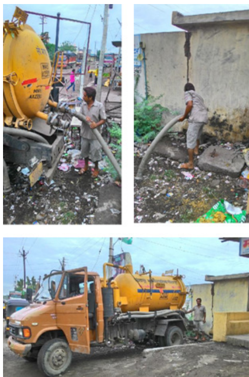
Figure 2: Emptying septic tank of community toilet (source: Rahul/CSE, 2015)
