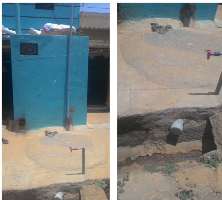
Figure 2: Toilet connected to a pit with opening for emptying septage (Source: Rahul/CSE, 2015)
