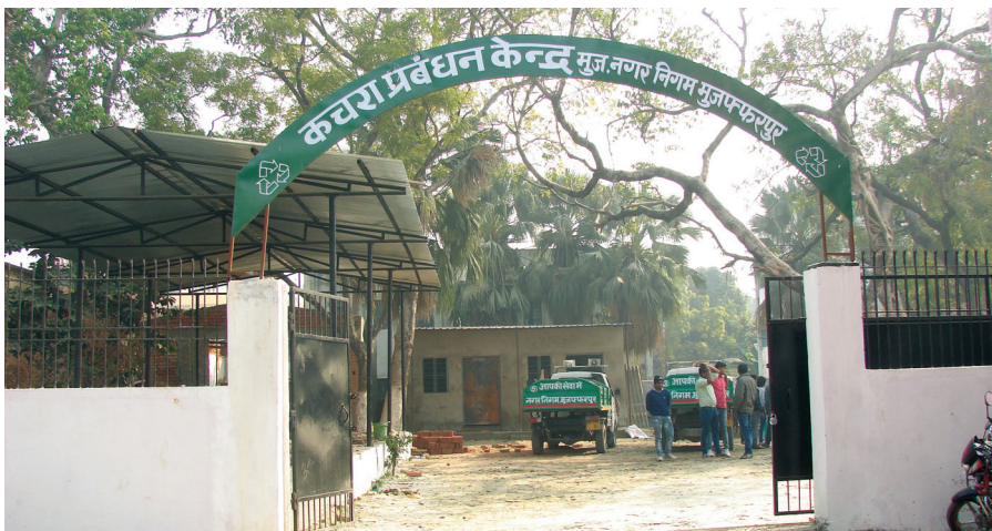
Model composting facility at the Town Hall
