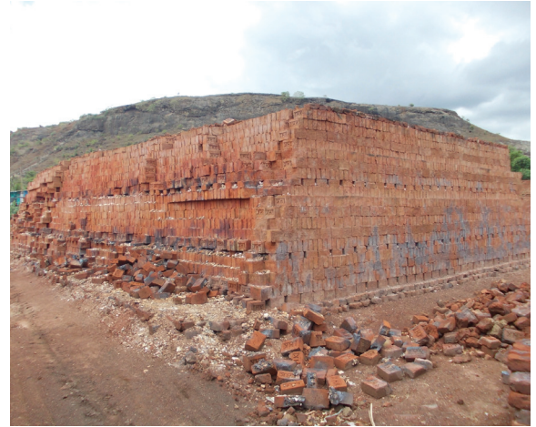
A typical clamp in the area producing around 3–4 lakh bricks per batch
