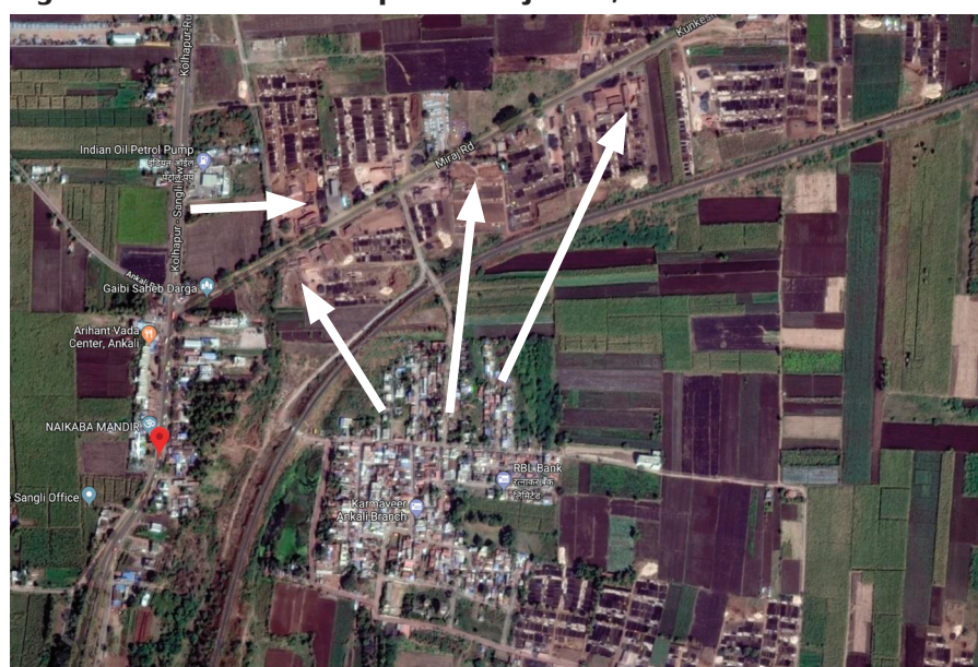
Figure 3: Location of clamps at Miraj Road, Ankali
