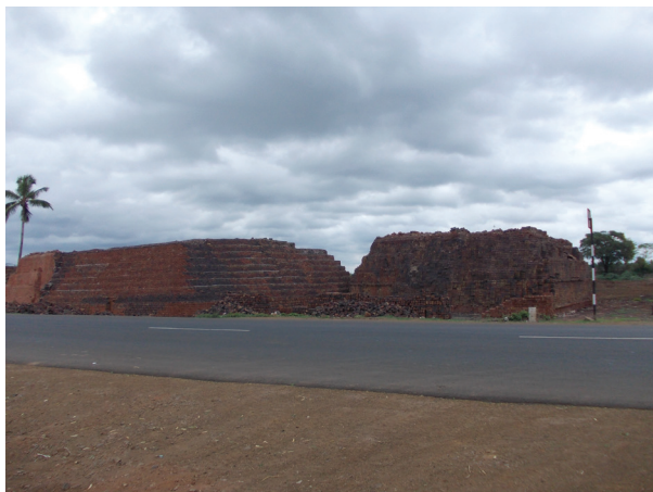
Clamps next to a road in Miraj Road, Ankali
