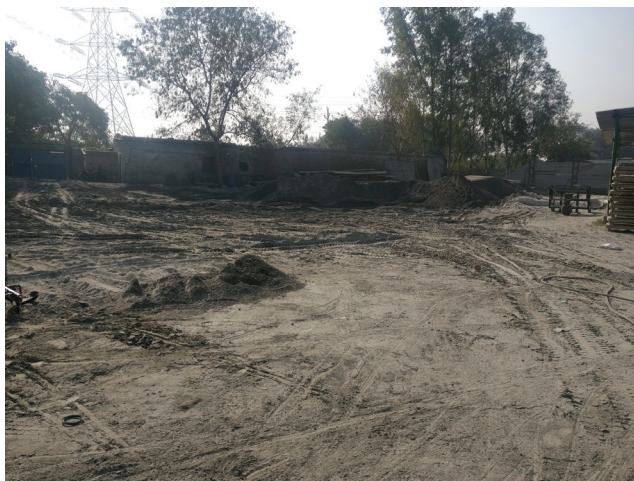
Fly ash littering within the premises of a unit at Dadri
