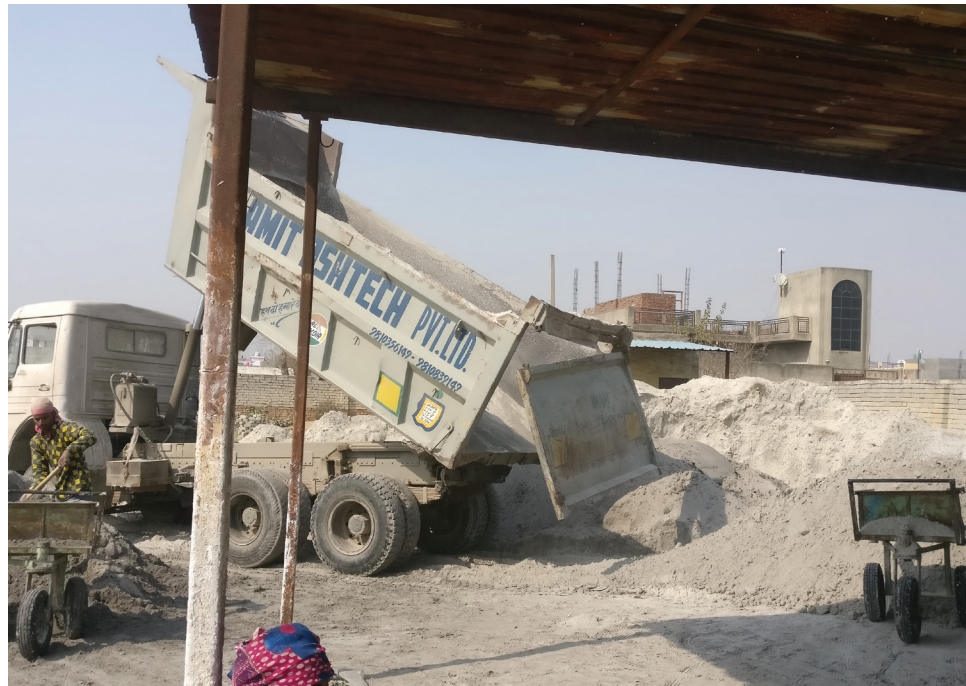
Unloading of fly ash at a unit in Ghaziabad
