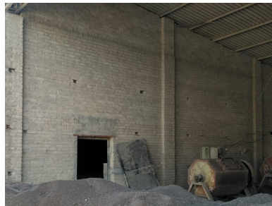
Side wall of the fly ash storage facility with a gate.
