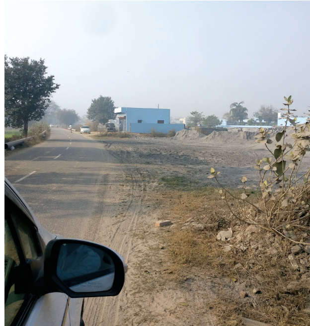
Fly ash littered on road due to the absence of boundary wall at plant in Gurugram
