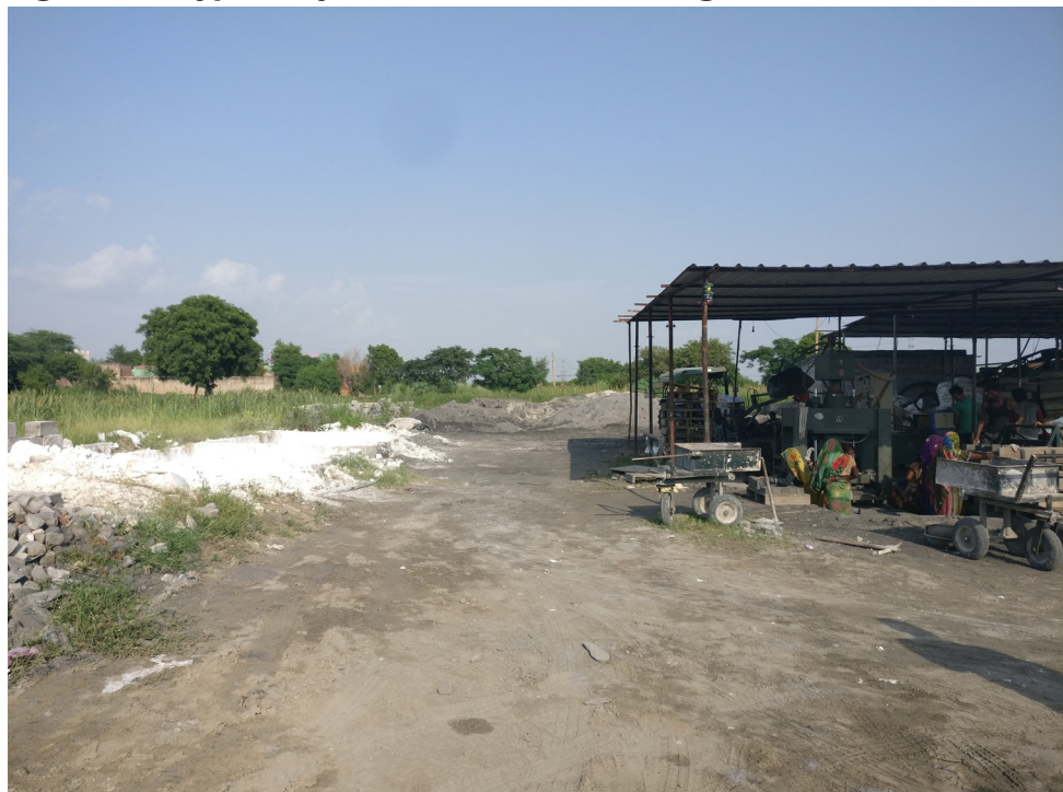
Figure 1: A typical fly ash brick manufacturing unit
