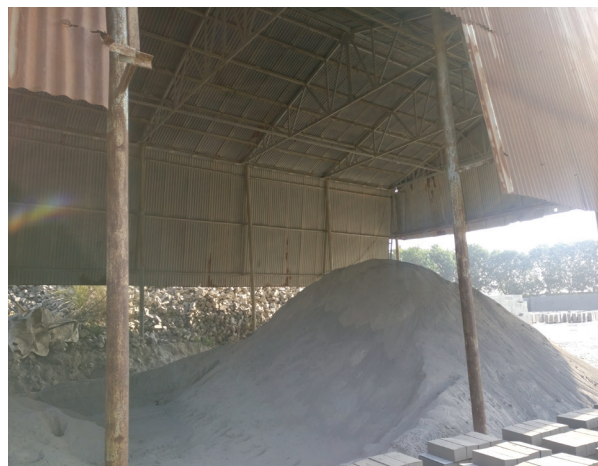
A make-shift storage facility in Delhi
