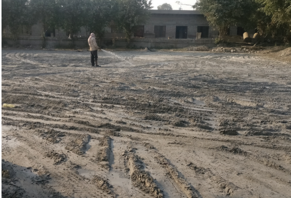
A unit at Dadri
