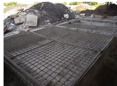
Covered lime ponds
