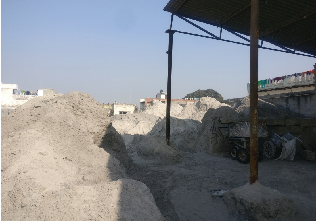
A fly ash unit next to a residential area in Dadri
