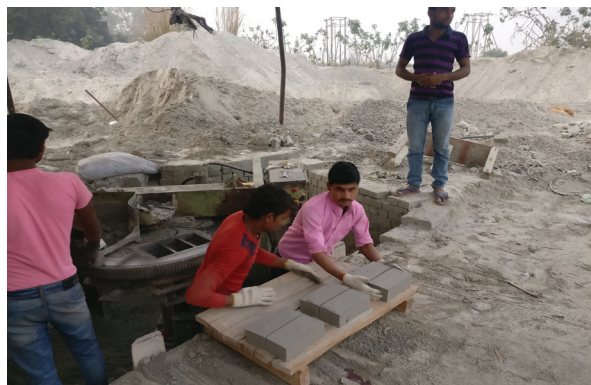
Workers using gloves at Deep Kamal Fly Ash, Greater Noida
