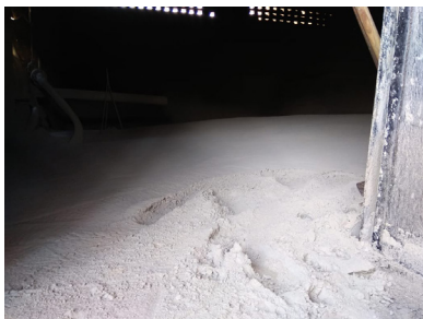
Inside of flyash storage facility
