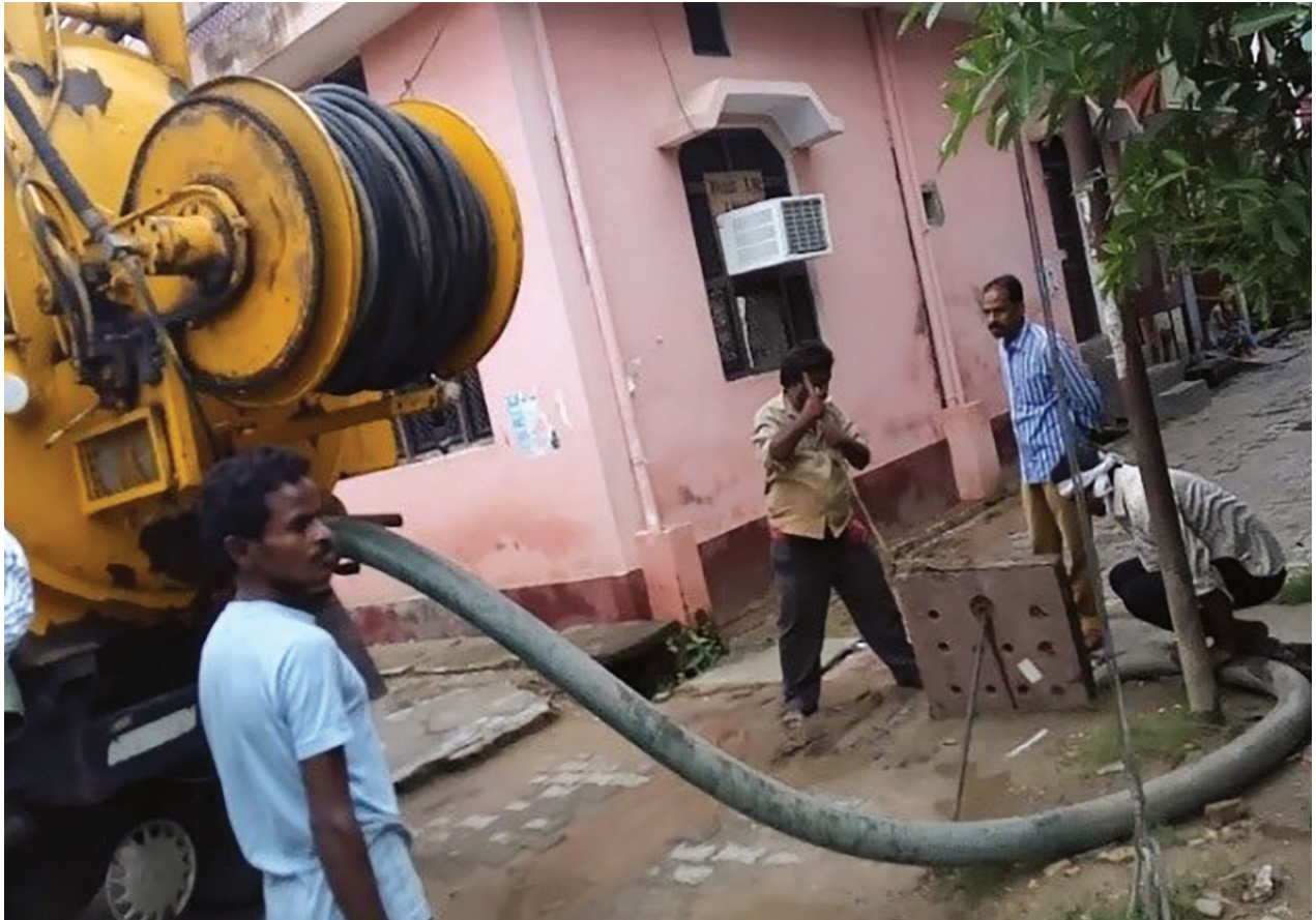
Mechanical emptying of containment system
