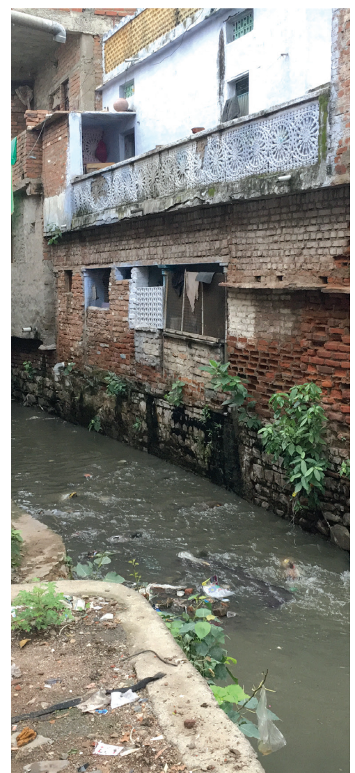
Household discharging wastewater directly into nullah
