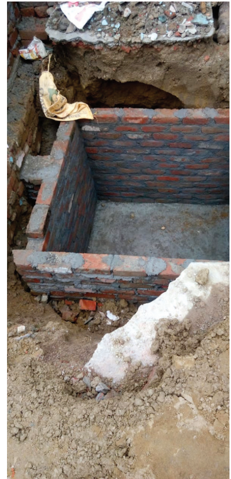
Fully lined tank under construction
