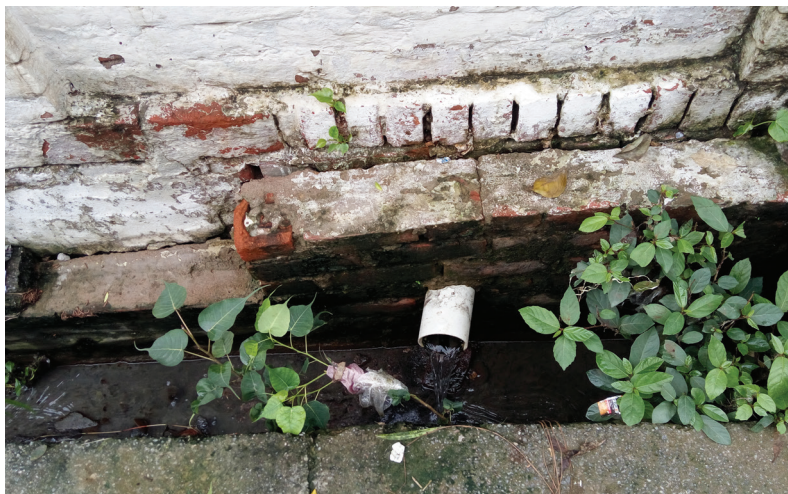
Outlet of a containment discharging into open drain
