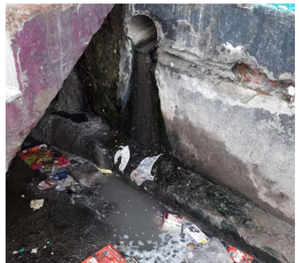
Figure 1: Supernatant of a tank discharges into open drain
