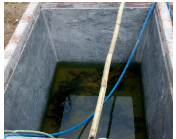
Figure 1: Septic tank of a household under construction
