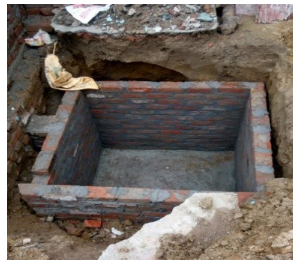
Figure 1: Fully lined tank under construction of a household
