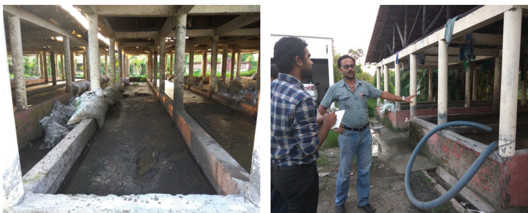
Figure 14: Sludge drying beds (Source: Aishwarya/CSE, 2016)
