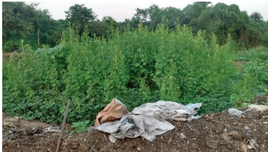
Figure 16: Visible plant growth after a year of rainfall (Source: Aishwarya/CSE, 2016)
