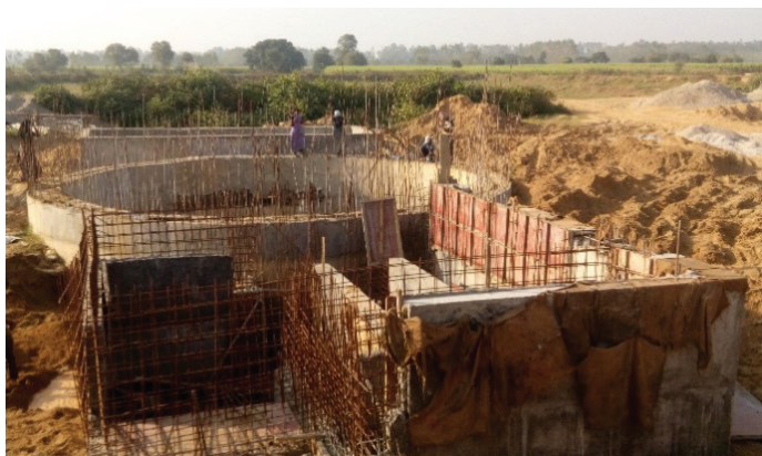
Figure 6: Screens, classifier and equalisation tank of STP under construction at Bijnor (Source: Amrita/CSE 2016)
