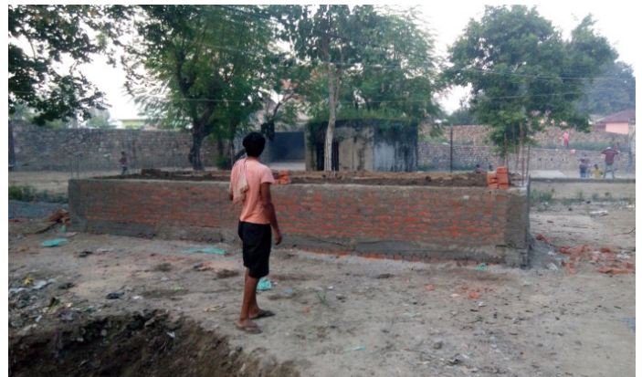
Figure 10: Under construction community toilet at Ramrekha Ghat (Source: Amrita/CSE, 2016)
