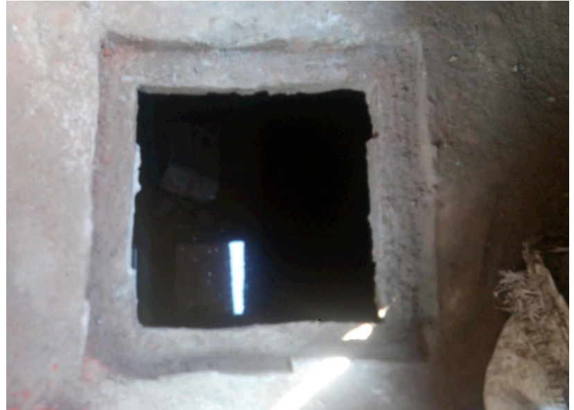
Figure 3: Newly constructed septic tank (Source: Amrita/CSE, 2016)
