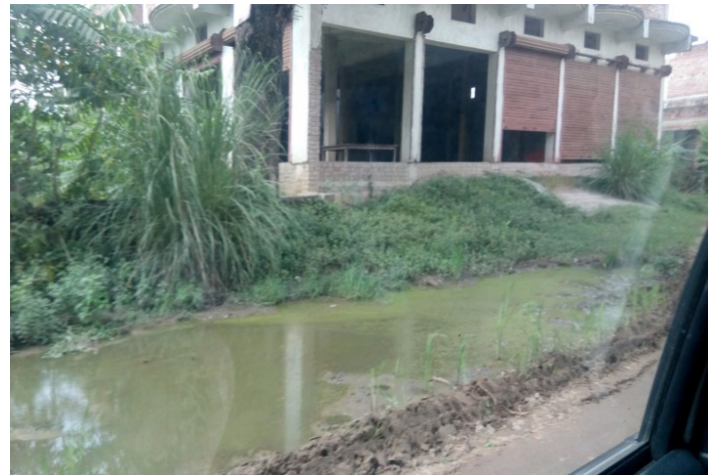
Figure 17: FS discharging spot (Source: Amrita/CSE, 2016)
