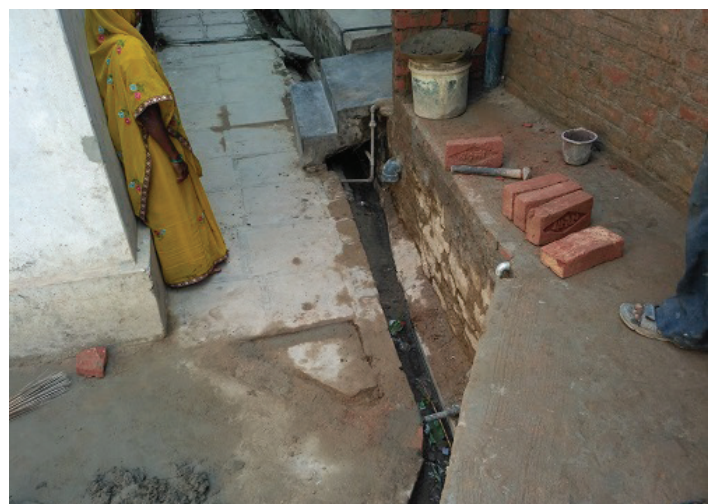
Figure 2: Septic tank with effluent pipe connected to open drain (Source: Shantanu/CSE, 2016)
