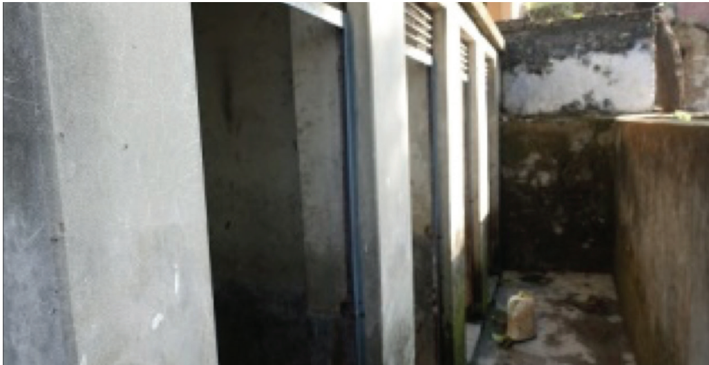
Figure 11: Community toilet at Balughat (Source: Shantanu/CSE, 2016)
