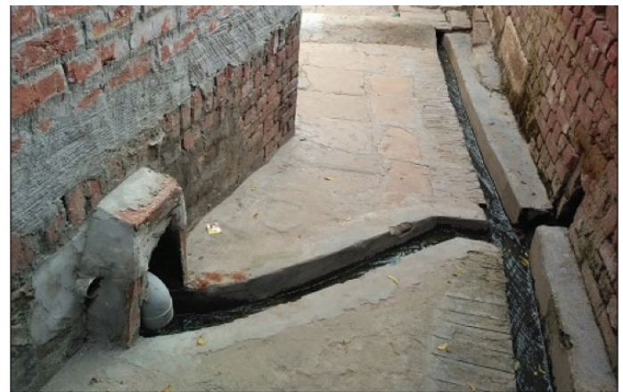
Figure 1: Septic tank connected to open drain (source: Bhavik/CSE, 2016)
