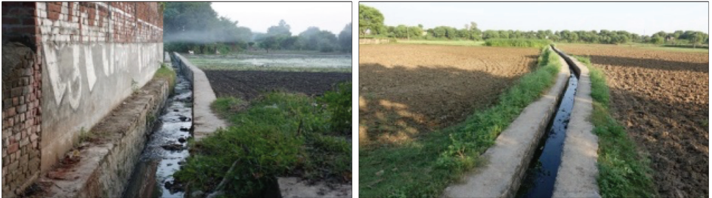
Figure 4: Nullahs discharging wastewater on agriculture fields (Source: Shantanu/CSE, 2016)
