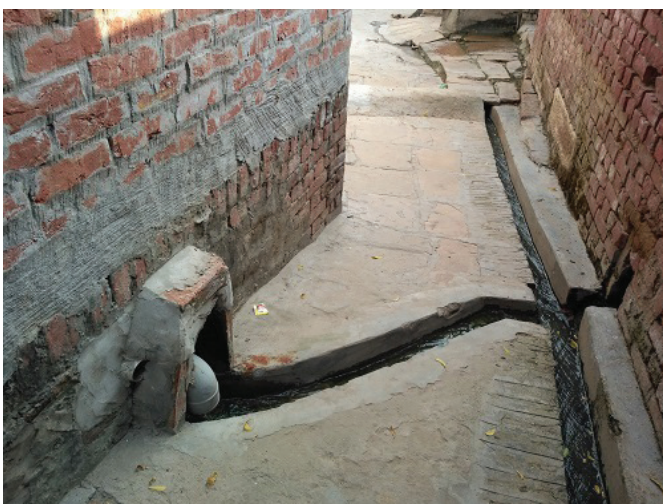
Figure 2: Septic tank with effluent pipe connected to open drain (Source: Shantanu/CSE, 2016)
