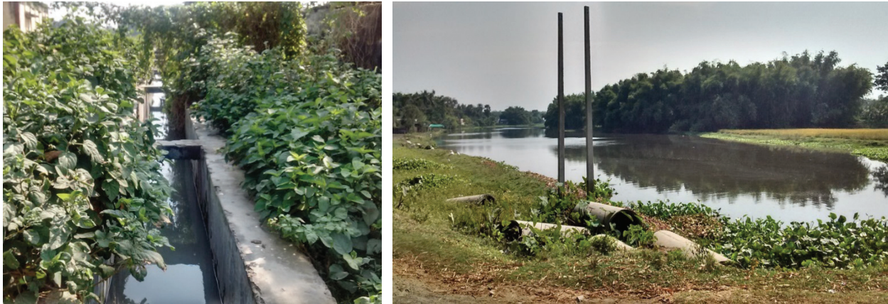
Figure 8: WW being drained out to low lying areas in ward 45 (Source: Anil/CSE, 2016)
