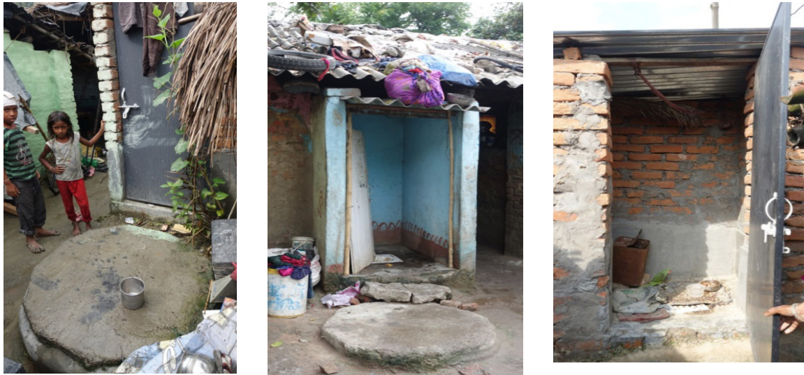
Figure 9: Toilets constructed under SBM connected to pit in slum (Source: Anil/CSE, 2016)
