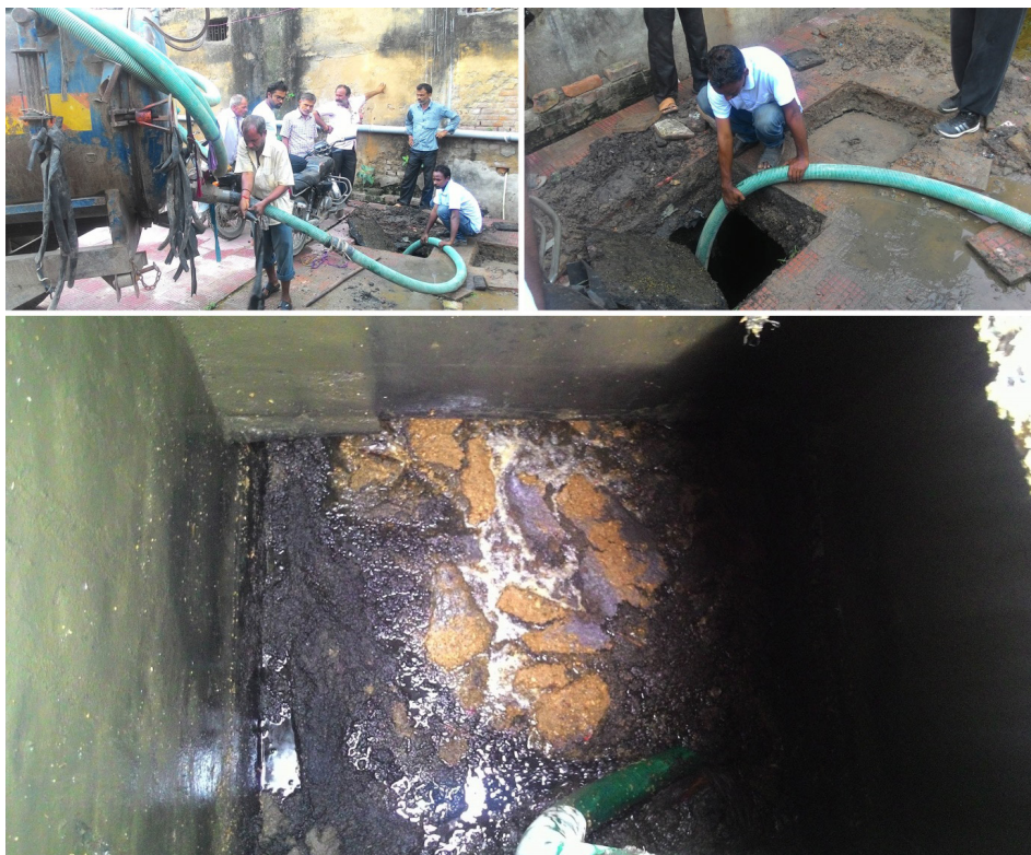
Figure 5: Emptying process of a septic tank (Source: Bhitush/CSE, 2016)
