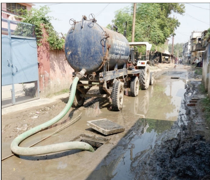
Figure 3: Vacuum tanker is used for unclogging sewer manholes (Source: Bhavik/CSE, 2016)
