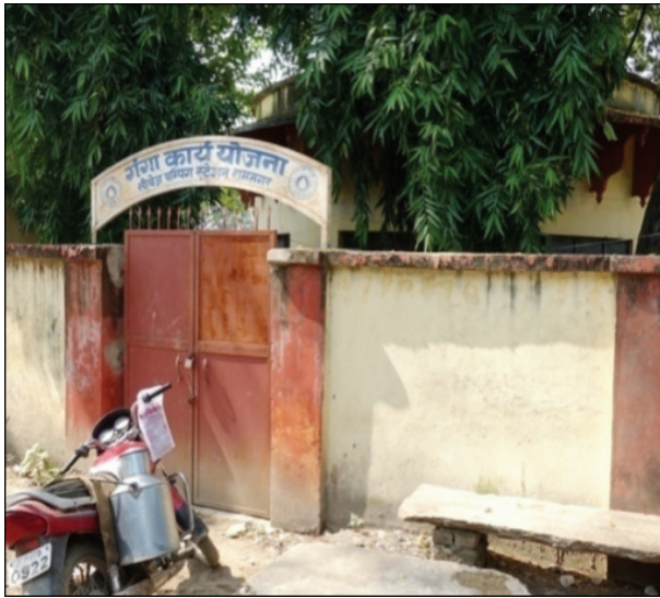
Sewage Pumping Station
