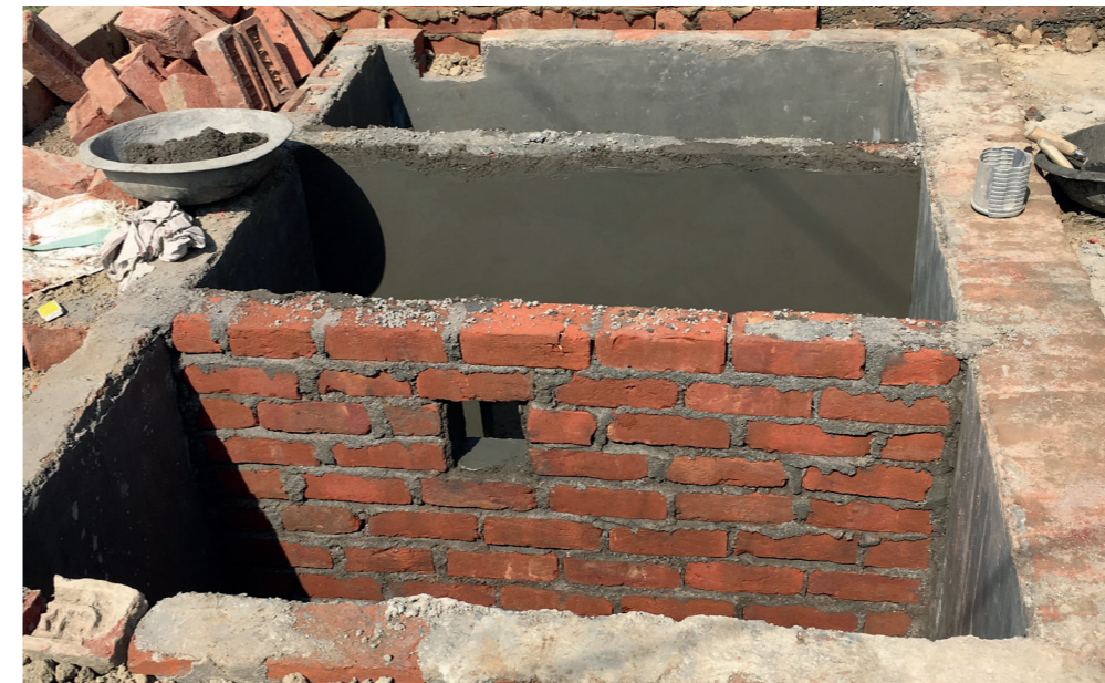
Septic tank under construction, Hardoi
