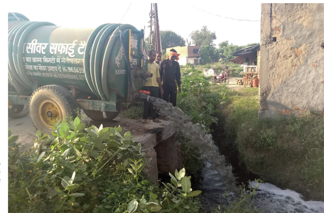
Faecal sludge discharged in open drain, Hathras
