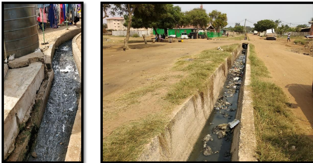
Figure 10: Open drain/storm water is also used to transport grey water (Shantanu/CSE, 2018)
