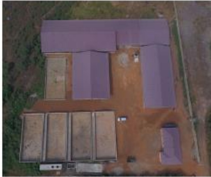
Figure 20: Birds eye view of the JVL treatment plant
