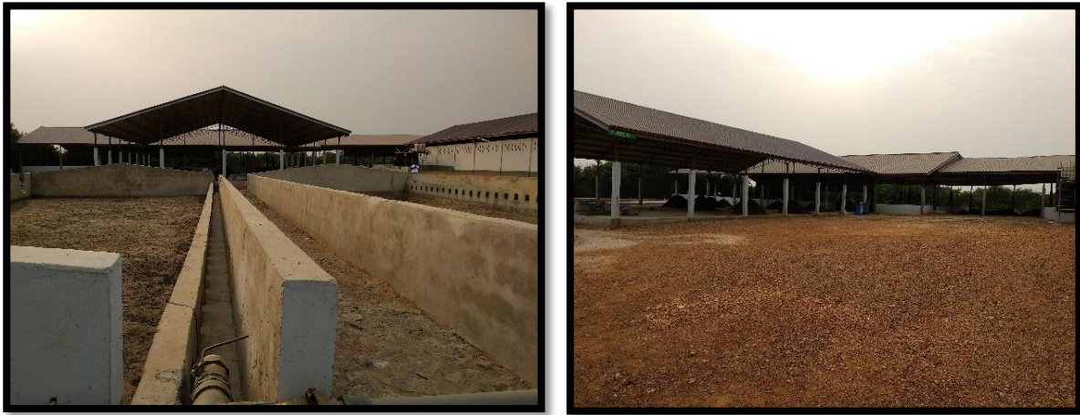
Figure 19: Septage treatment facility – a co composting plant at Bortyemen
