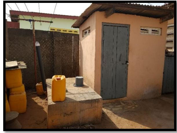
Figure 5: Toilet constructed under scheme with fully lined tank (Amrita/CSE, 2018)
