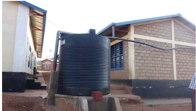
Plastic tank used for storage constructed above ground
