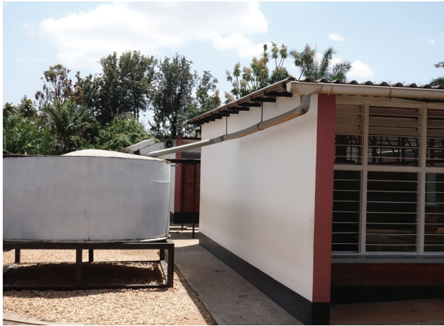
Masonry tank used for storage constructed above ground
