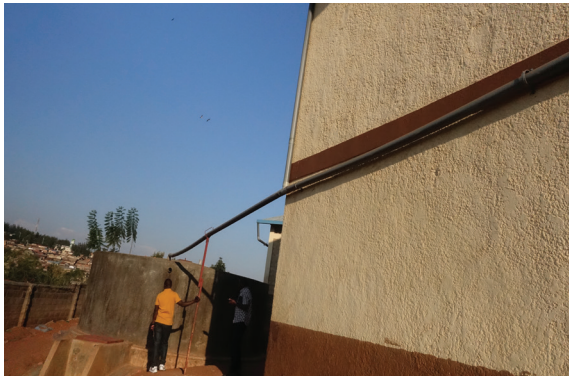
Masonry tank used for storage constructed above ground
