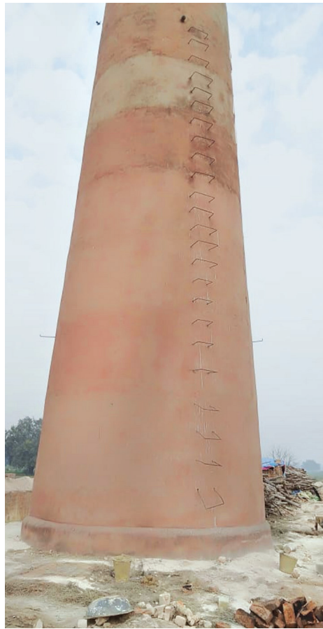
Figure 2: Monkey ladder without platform. (Kanpur, UP; 21-Feb-2019)
