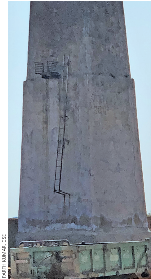
Figure 1: Ladder provided 6 feet above ground (Bharatpur, Rajasthan; 19-Mar-2019)
